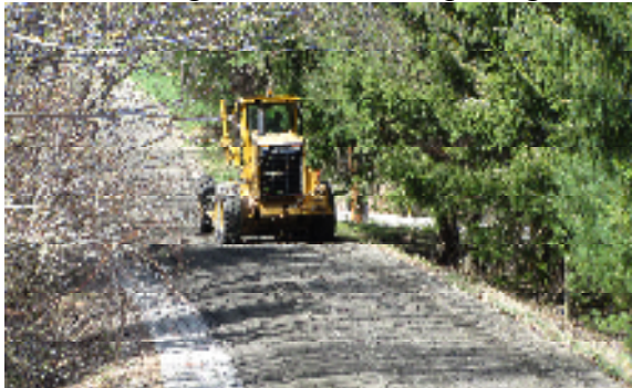
Grading Nichols Hill for paving:
